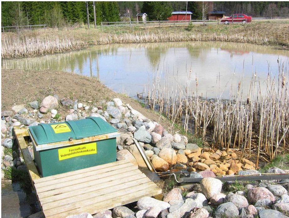
Fig. 6. A Ferrix-dozer and a settling pond in Lake Rehtijärvi area, Jokioinen. At this site, ferric sulphate was dozed during spring flood, and application of 400 kg of Ferrix-3 stripped 1 kg of P from water containing 60–140 \mu\text{g DRP l}^{-1} (i.e., typical field runoff situation); in hot-spot ditches, a higher efficiency is obtained.
