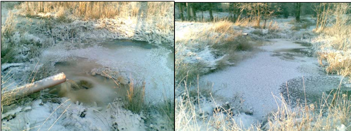
Figure 11. Sedimentation pond in winter.
